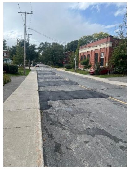
3- 2024-10-01 Fresh repairs on Curzon
